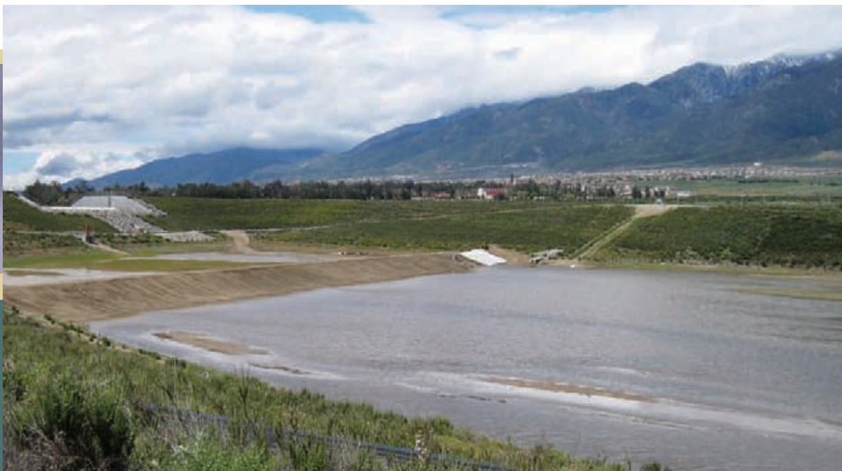
San Sevaine Recharge Basin following a winter storm.
