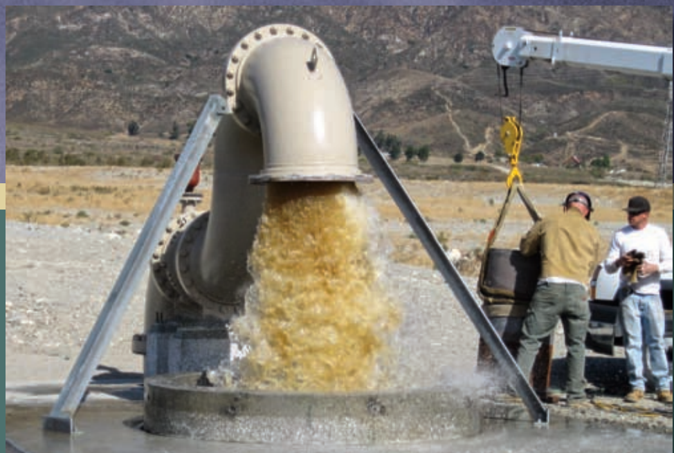
Purging of the improved MWD connection CB-14.
