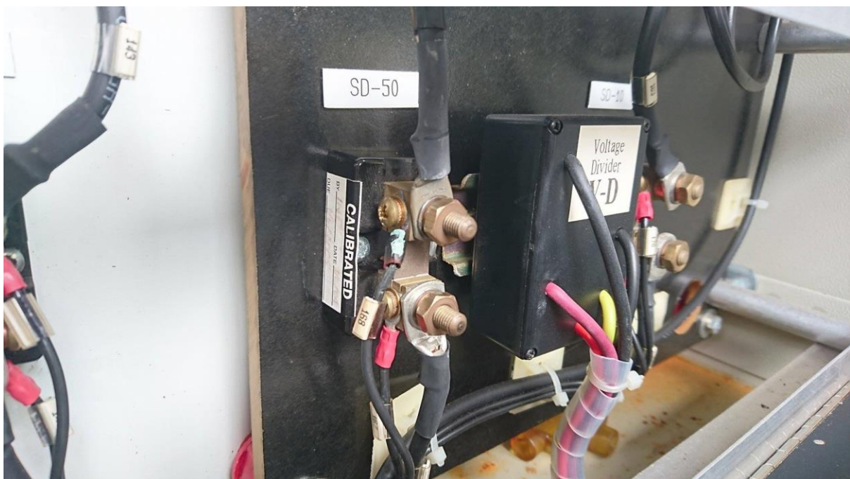
Figure 23: Newly Installed Current Shunt
