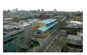
This image shows an aerial view of St. John's Wood 400kV substation in north London. Amongst other factors, design of this GIS (gas insulated switchgear) substation had to take into account land constraints in this urban area.
