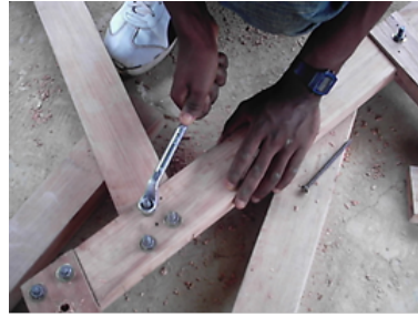
Figure 4: Fastening with bolts and nuts
