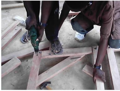
Figure 3: Drilling holes for bolts and nuts
