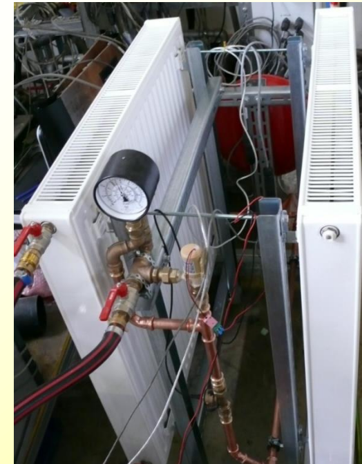
TEG cooling system
