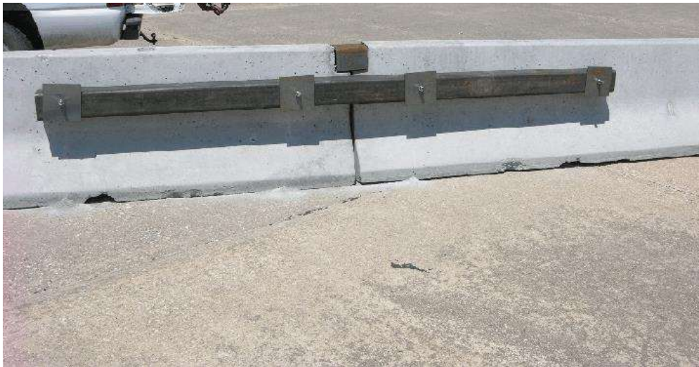
Figure 25. NYSDOT Box-Beam Stiffener System [29]
