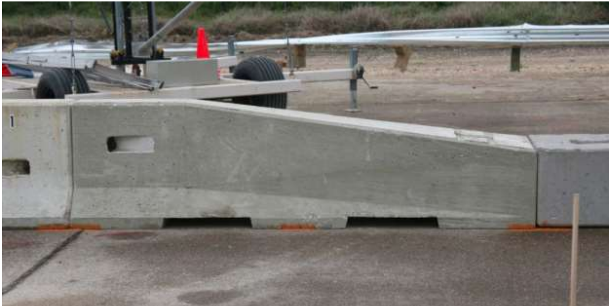
Figure 22. Low-Profile-to-F-Shape Transition Barrier Segment [25]
