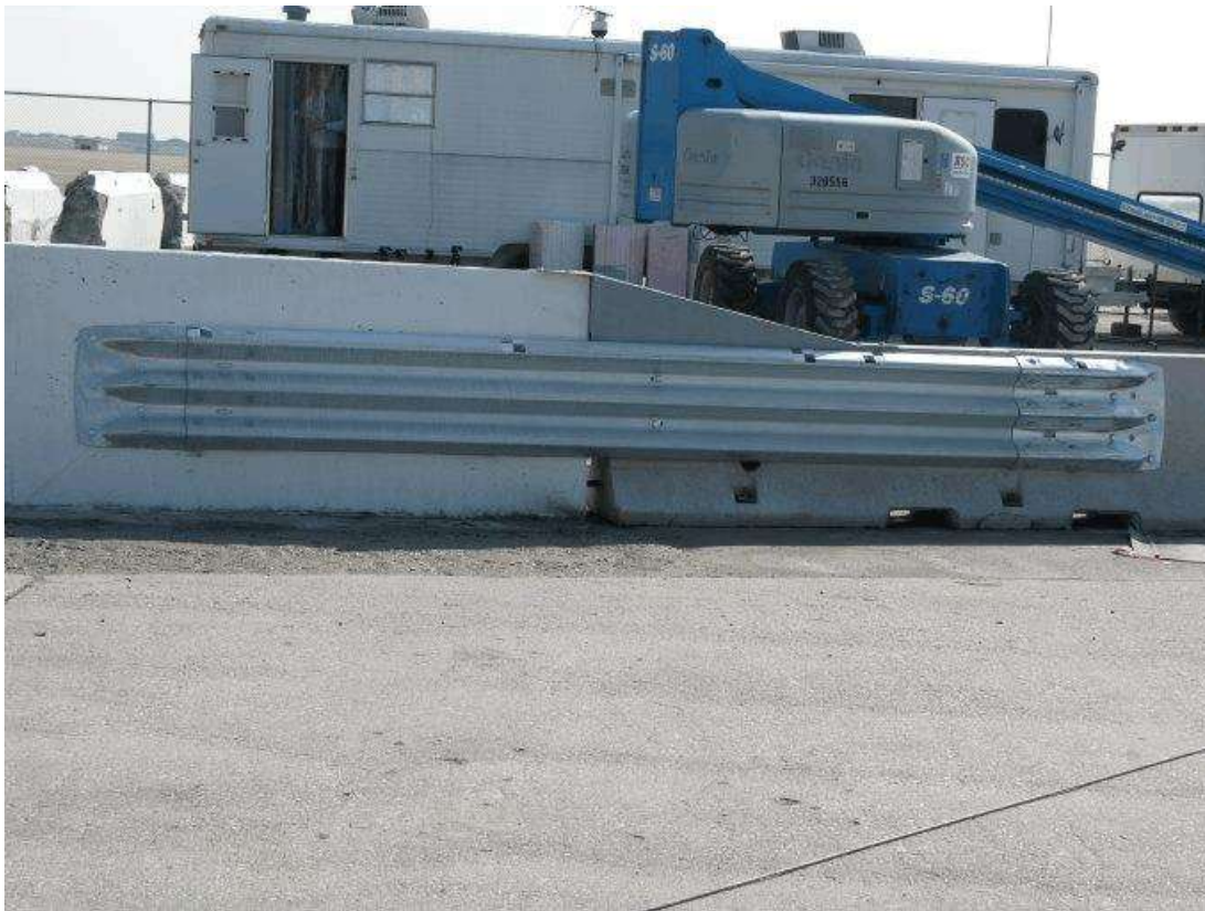
Figure 11. Transition from PCB to Permanent Concrete Barrier [2]
