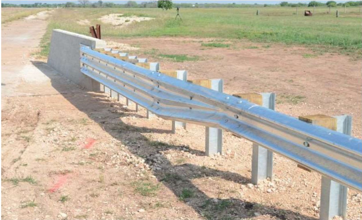
Figure 20. Thrie Beam Transition without Curb [23]
