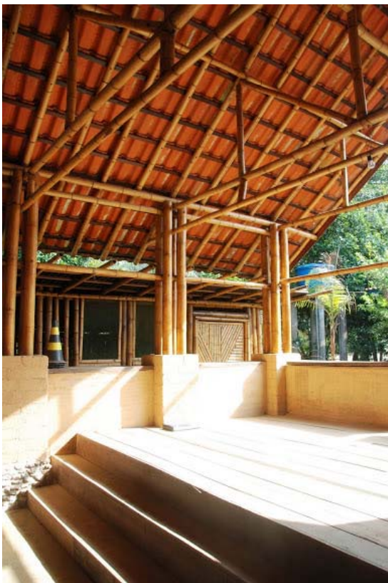
a) Community center with overbuilt columns and roofing system.
