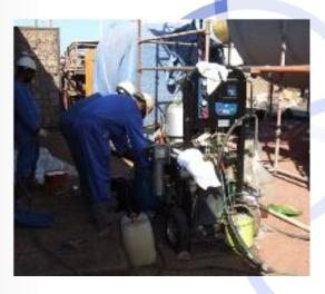
Dual Component Heated Airless Spray
