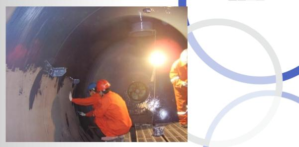
• Used for the internal lining of process vessels Subject to erosion and corrosion from aggressive fluids.
