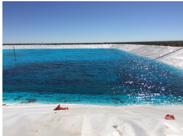
Freshwater Hydro Testing New Impoundment
