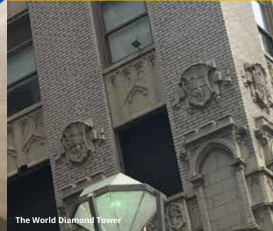
Lobby Renovation: 580 Fifth Avenue
