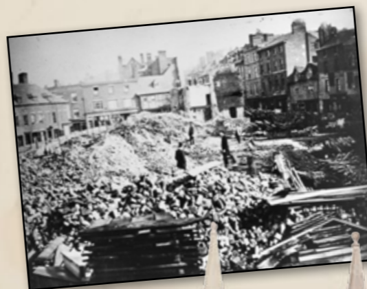
Buildings demolished to make way for the New Market Hall, Clarendon Street, Shrewsbury, c. 1866. Shropshire Archives ref. PH/S/13/C/18/9
