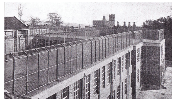
Pendower School, with its distinctive roof playground
