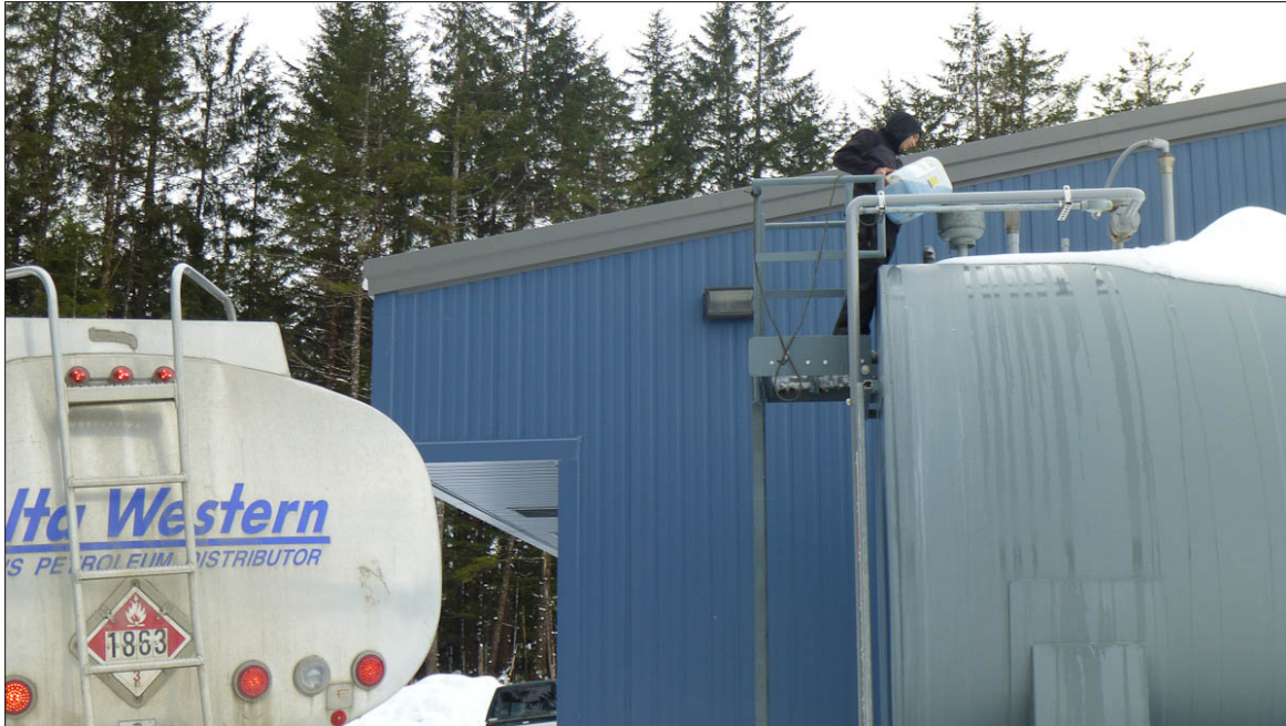
Figure 13. "Splash blending" of an additive at the Yakutat Power for testing purposes. Note fuel truck delivering fuel to the power plant and the worker adding a liquid to the tank during fuel delivery, using the mixing provided by the fuel movement during transfer to mix the additive with the fuel. Photo by Scott Newlun.
