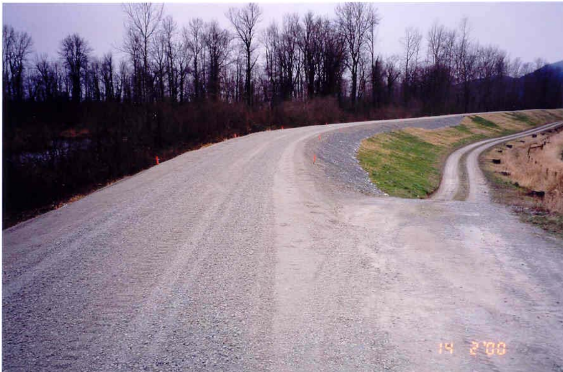
Photograph 4: Access Ramp and Turnout
