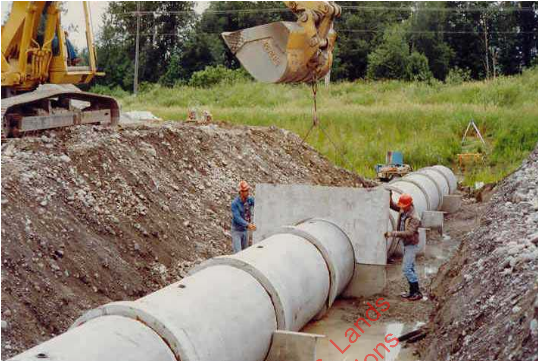
Photograph 23: Cutoff Wall Installation
