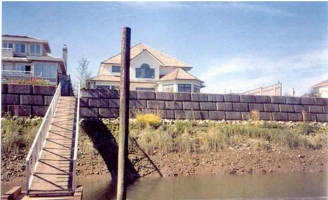
Photograph 21: Lock Block Retaining Wall with Gangway to Float
