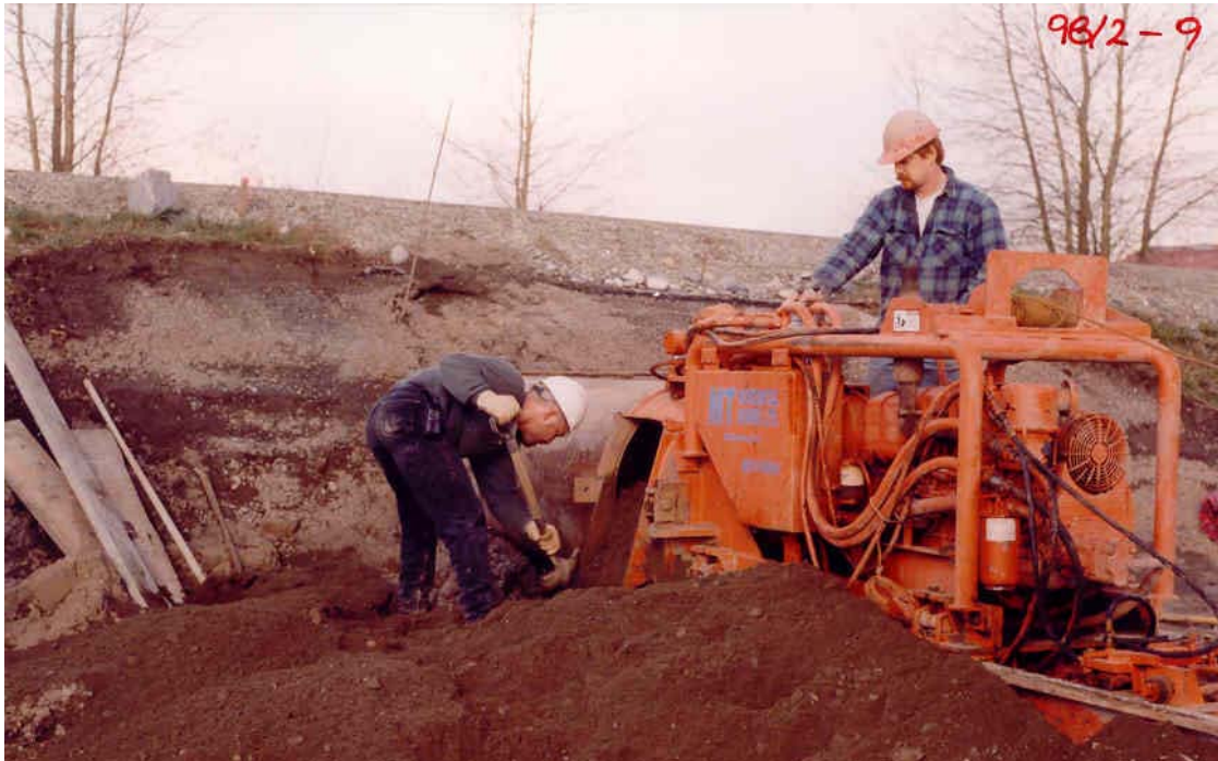
Photograph 26: Pipe Jacking
