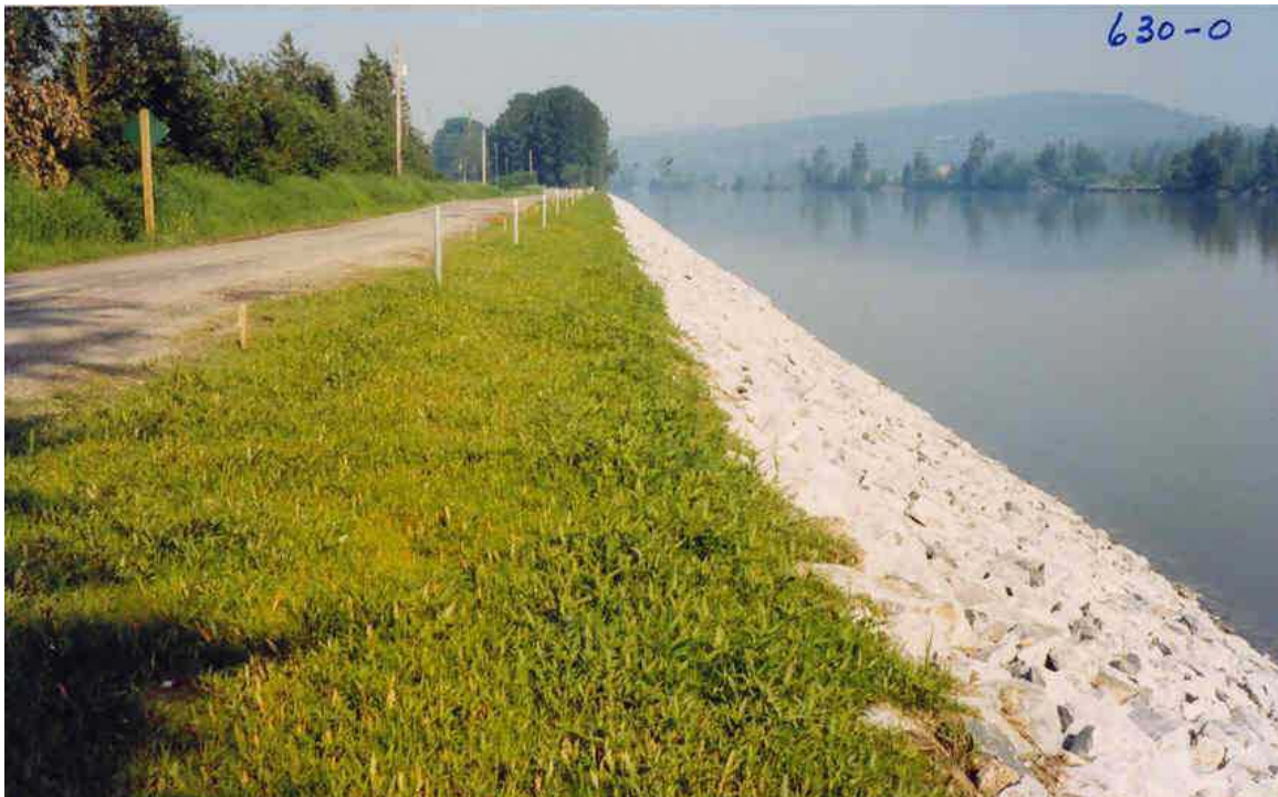
Photograph 14: Rock Riprap Erosion Protection
