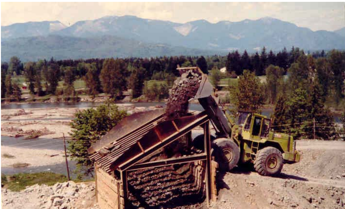
Photograph 13: Grizzly For Production of Dike Materials
