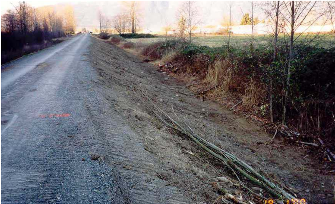
Photograph 30: Site Preparation Prior to Dike Upgrade
