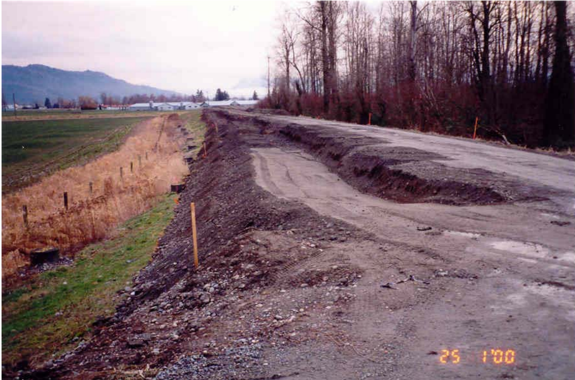
Photograph 12: Drainage Layer and Pressure Relief Wells
