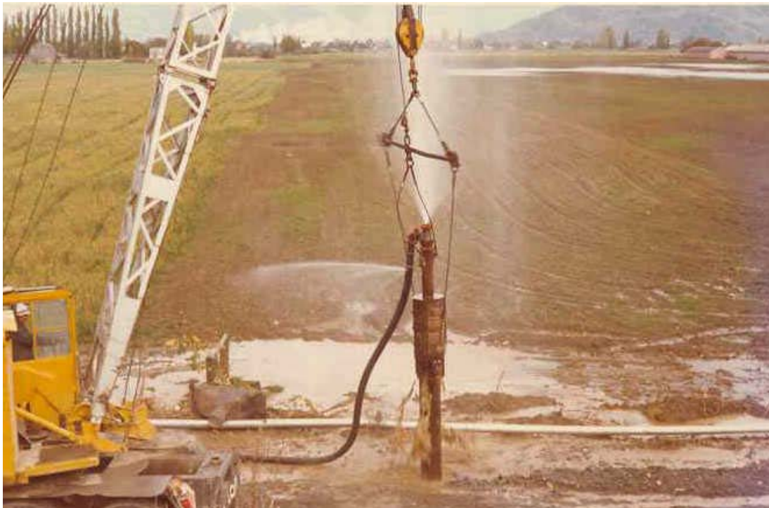
Photograph 10: Installation of Pressure Relief Wells
