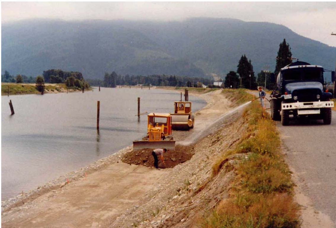
Photograph 34: Water Placement For Optimum Soil Moisture
