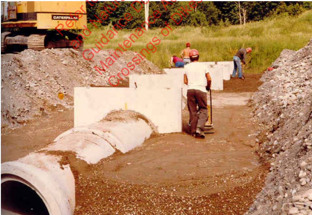
Photograph 24: Cutoff Wall Installation
