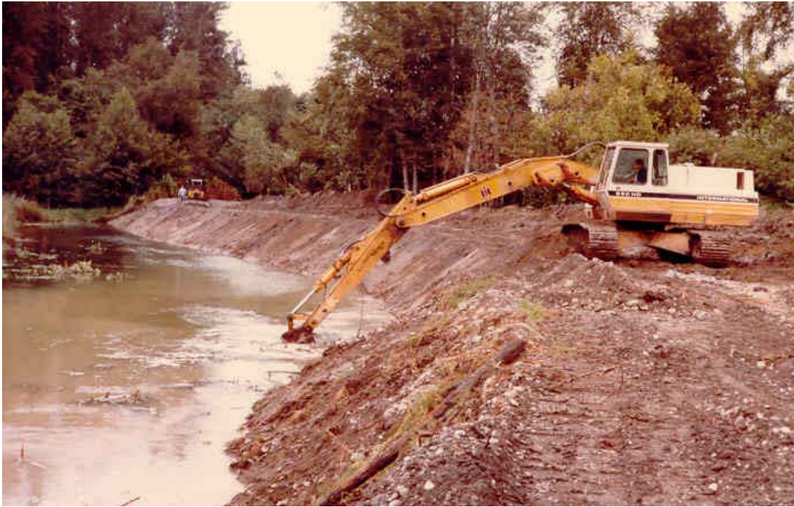
Photograph 11: Flattening Sideslopes to Install Impervious Layer
