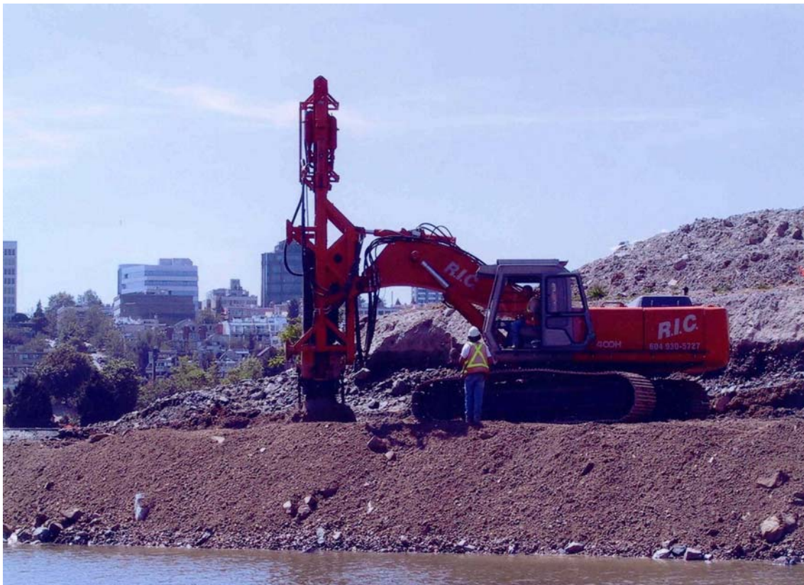
Photograph 35: Rapid Impact Compaction
