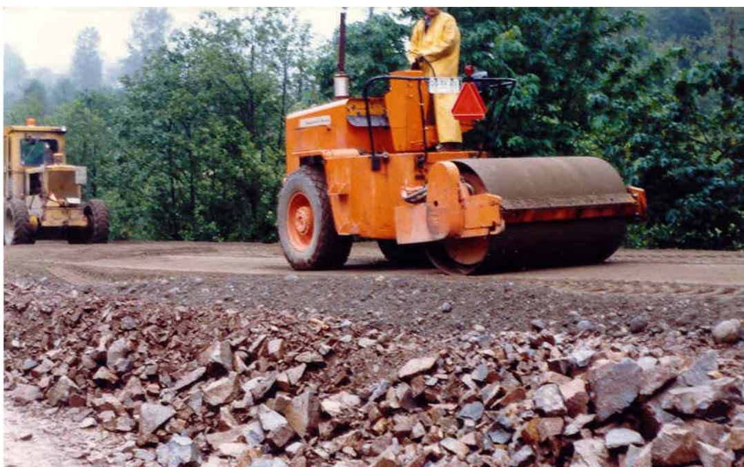
Photograph 32: Vibratory Roller
