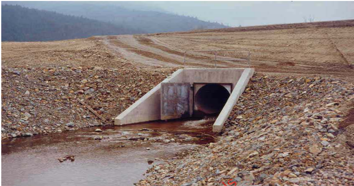
Photograph 17: Headwall With Wingwalls and Flapgate
