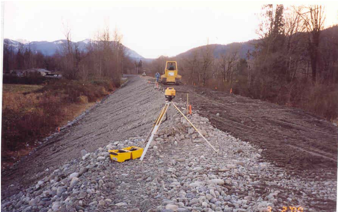
Photograph 31: Survey Layout For Dike Upgrading
