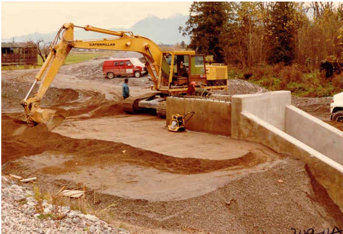
Photograph 18: Compaction of Dike Materials Adjacent to Structures
