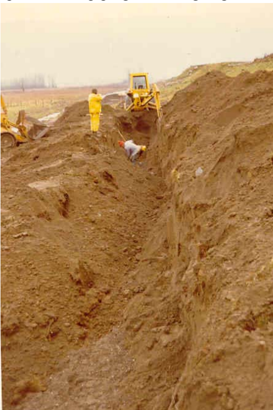
Photograph 8 Installation of Pervious Toe Trench
