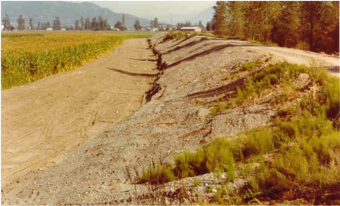
Photograph 7: Construction of a Landside Seepage Berm
