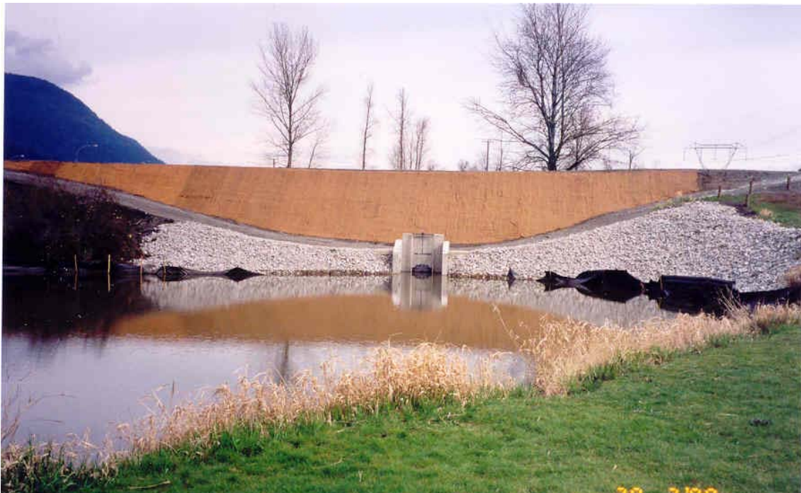
Photograph 29: Bank Protection on Outlet Side of Dike
