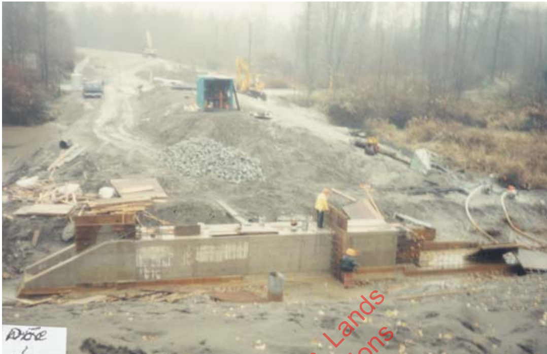
Photograph 25: Transverse Pipe Crossing
