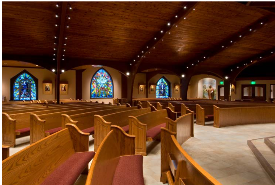
Figure 9. View of Hudson River valley worship space, showing track mounted to beams with MR16 track heads aimed downward into pews. (Foresight Architects, Schenectady N.Y.; Randall Perry Photography, Schaghticoke N.Y.)
