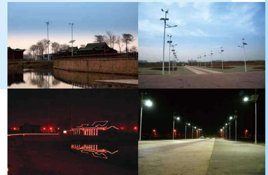
Zhongwei City, Ningxia wind & solar hybrid landscape lighting system 2011
