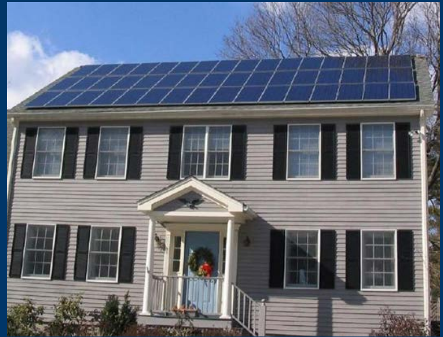
Solar panels on roof
