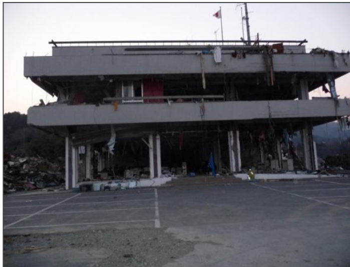
Town hall in Onagawa Town, Miyagi Prefecture
