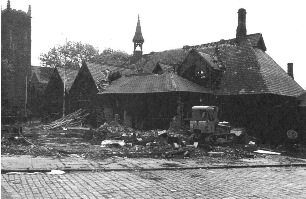
War damage, St Paul's CofE School, Great Portwood Street, Stockport. An example of the work needing doing after World War II.
