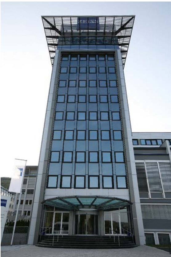
To frame the complete building the camera had to be tilted upwards. Converging vertical lines are then a natural consequence and no lens aberration.
