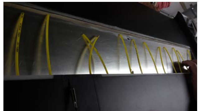
Fig. 14 – View of cooling system
