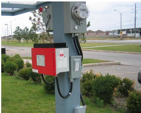
2. **Grid-tied** inverter systems use the utility as a “storage battery” by delivering excess energy to the distribution system, and consuming energy from the utility when DG output is lower than energy needs.
