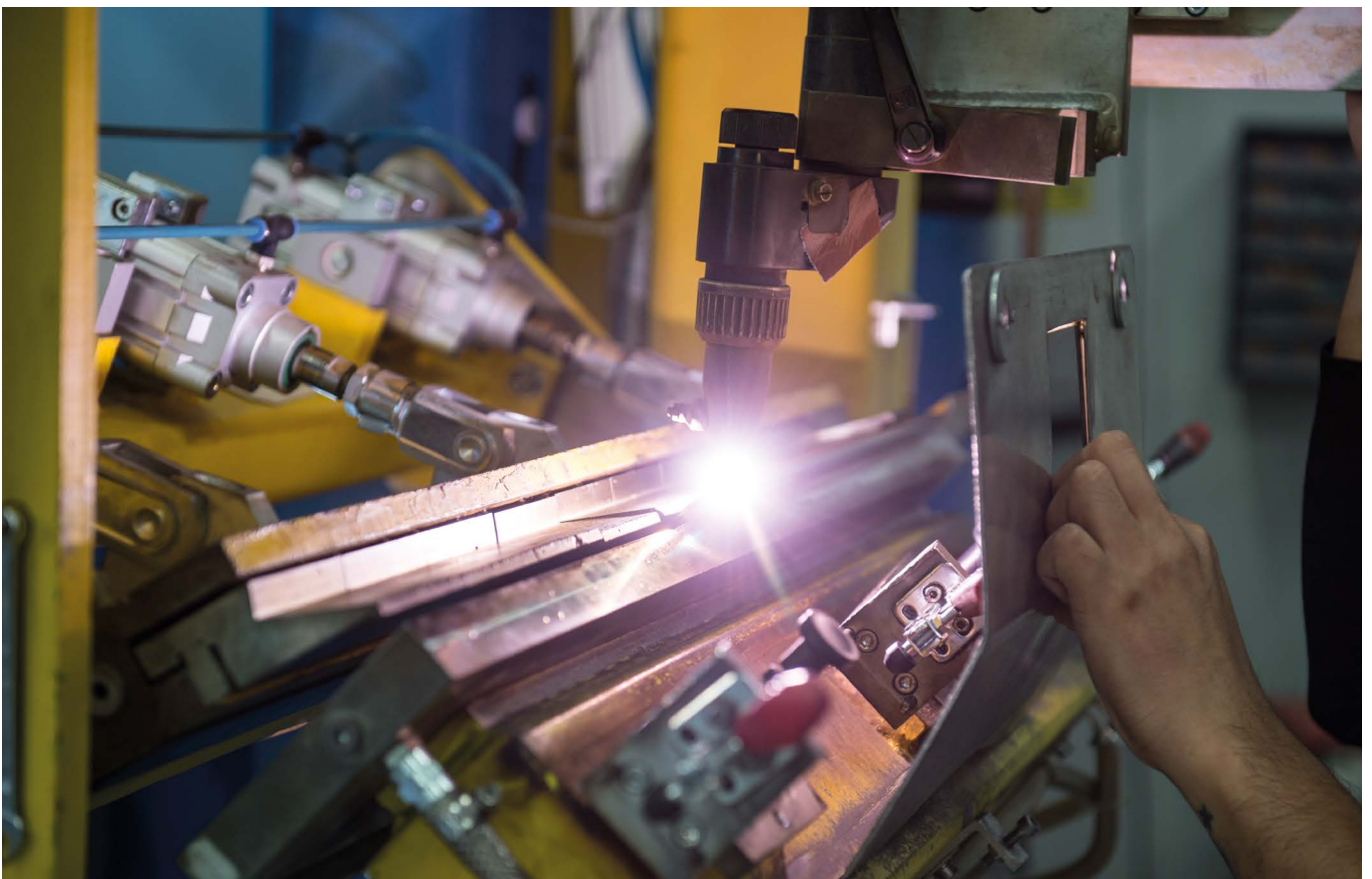
Welding the low-voltage connection of the secondary coil
