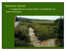
Connecting impervious surfaces with natural streams, roadside ditches influence the sediment loads, hydrologic regime, and quality of surface runoff. However, the extent and types of ditches have not been mapped in most watersheds.
