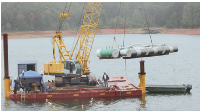
Johnson Offshore Intake Systems™ (JOIS™) Installation
