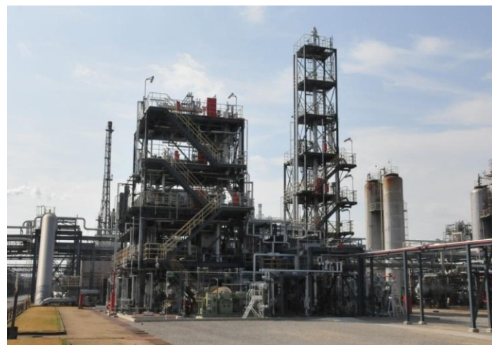
Demonstration Plant in Mizushima
