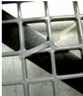
Attach Shorter Cable Ties to Corners
