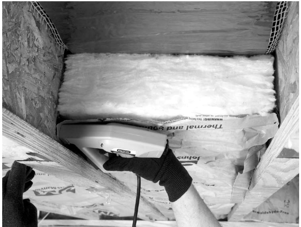
The mat power leads and sensor wire connected to the control at the electrical box.
