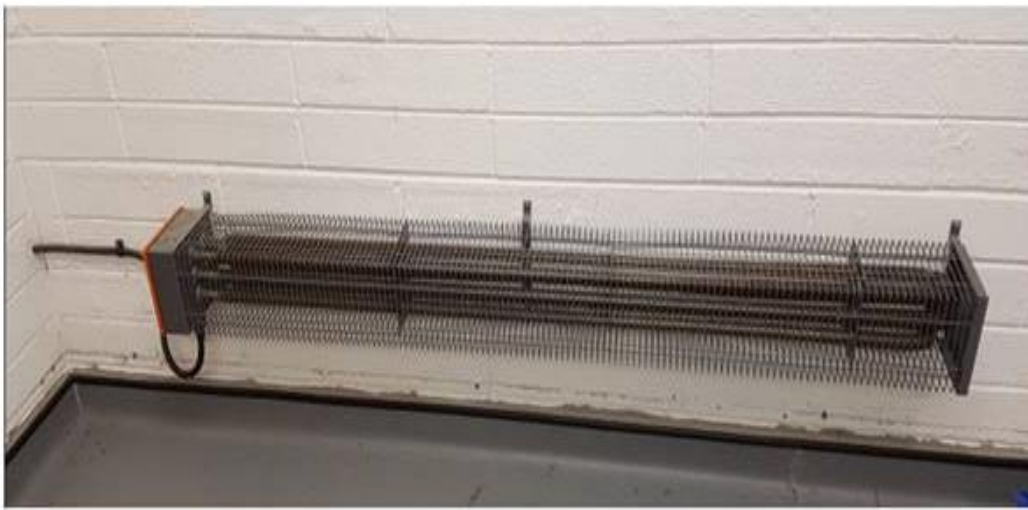
Figure 6 – Example cable wiring to Ex heater
