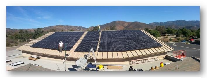
The **Pala Band of Mission Indians (CA**) installed a 91 kW solar system on their Fire Station which will save \$52,000 each year or \$1.3 million over the life of the system (May 2016)
