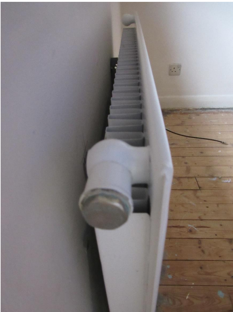
Figure 51 - A type 11 radiator.
