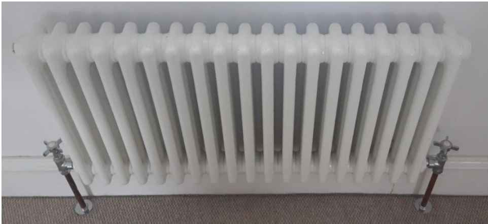
Figure 8 - A column radiator.
