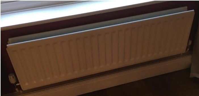
Figure 6 - A double panel radiator.
