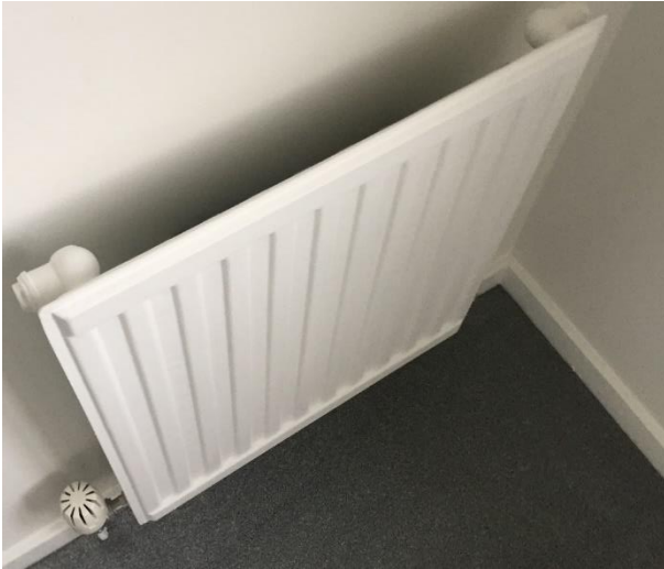
Figure 5 - A single panel radiator 33 .
