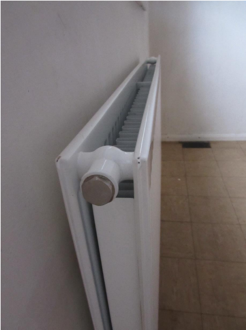
Figure 52 - A type 21 radiator.
