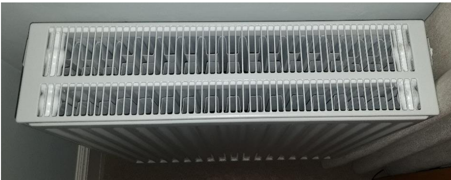
Figure 7 - A triple panel radiator.
