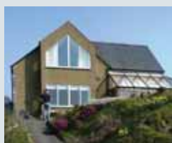
Domestic house West Wales
