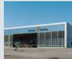
Ameco A380 Hangar, Beijing, China
