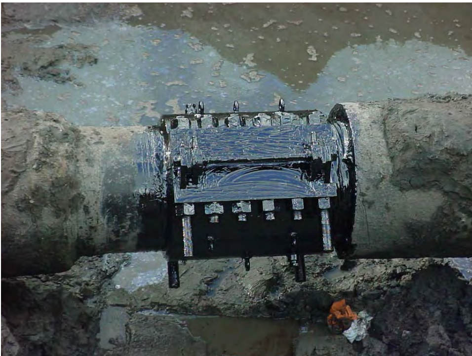
Figure 2 Installed PLIDCO sleeve at leak site MP 28
