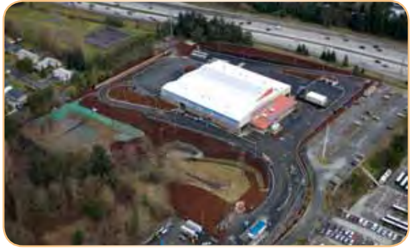
The new Shoreline Recycling and Transfer Station is fully enclosed to mitigate any potential impacts from noise, odor, and dust.
