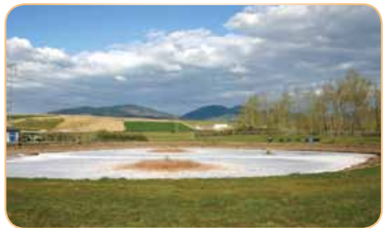
Leachate from the landfill is pretreated in an aeration pond before being sent to a wastewater treatment plant.
