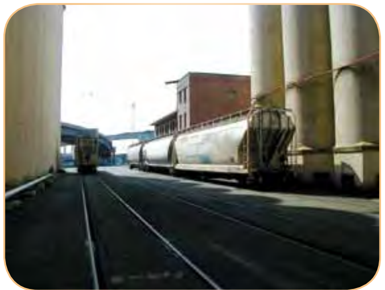
The Harbor Island property has access to the region's two rail lines.
