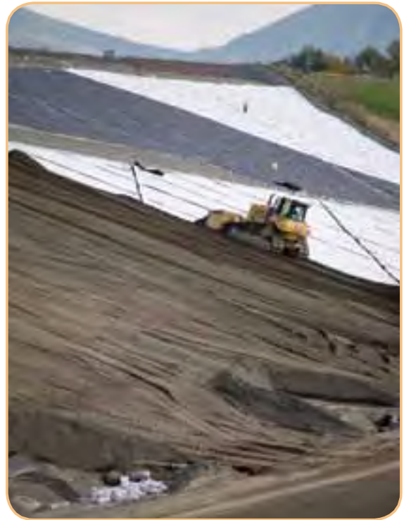
Portions of Area 6 are being prepared for closure with the placement of a soil and geosynthetic layer over the garbage.
