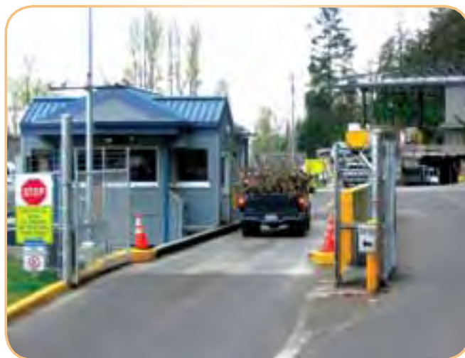
The Algona Transfer Station is one of five urban stations evaluated in the Transfer Plan.
