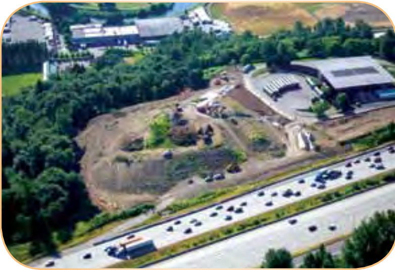
Site preparations are underway for constructing the new Bow Lake Transfer Station on property just north of the existing station.
