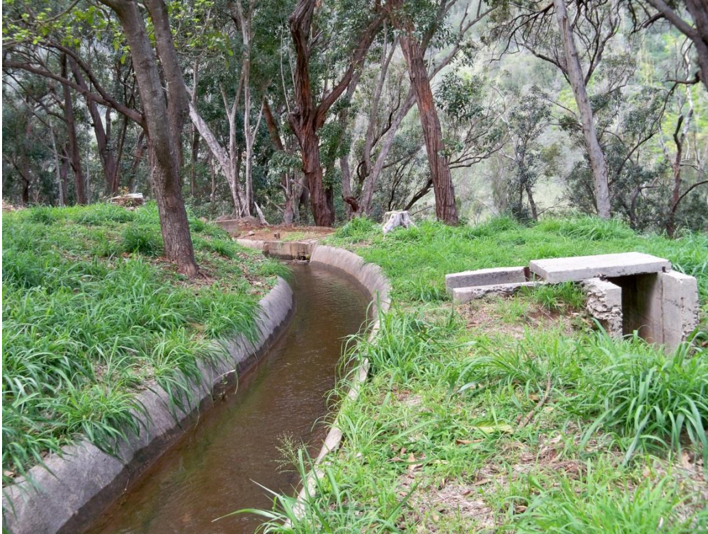
Figure 36. Photograph of Site 7881 Feature 1-Ditch (left) and Feature 6-Water Diversion (right) (View to North)
