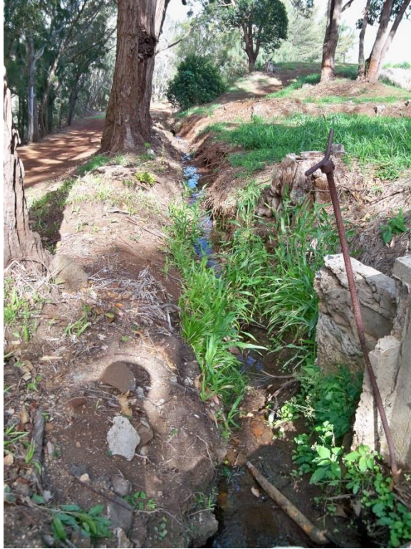
Figure 27. Site 7881 Feature 2 Ditch with Feature 5 in the foreground right (View to West)
