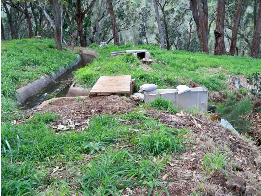
Figure 30. Overview Photograph of Feature 1 (Left) and Feature 3a (Right)
