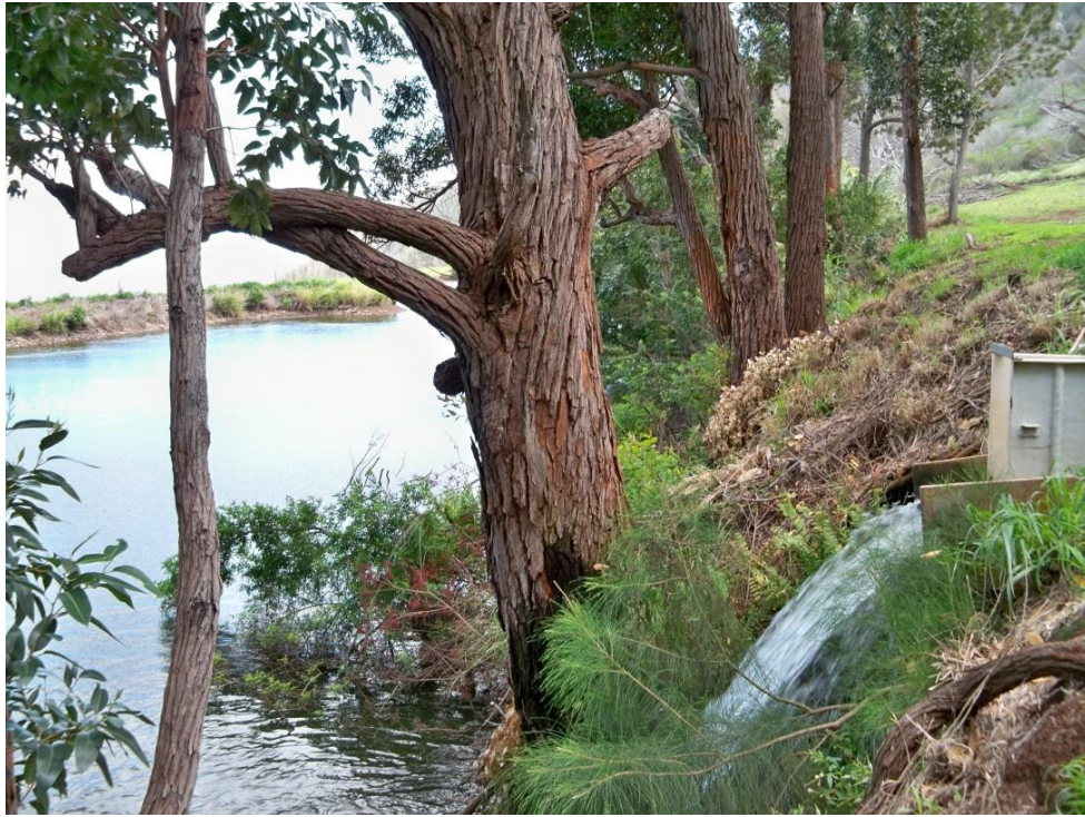
Figure 26. Site 7881 Feature 1 (TS1) Emptying into Reservoir (Feature 3) thru modernized Chute (Feature 3a) (View to South)
