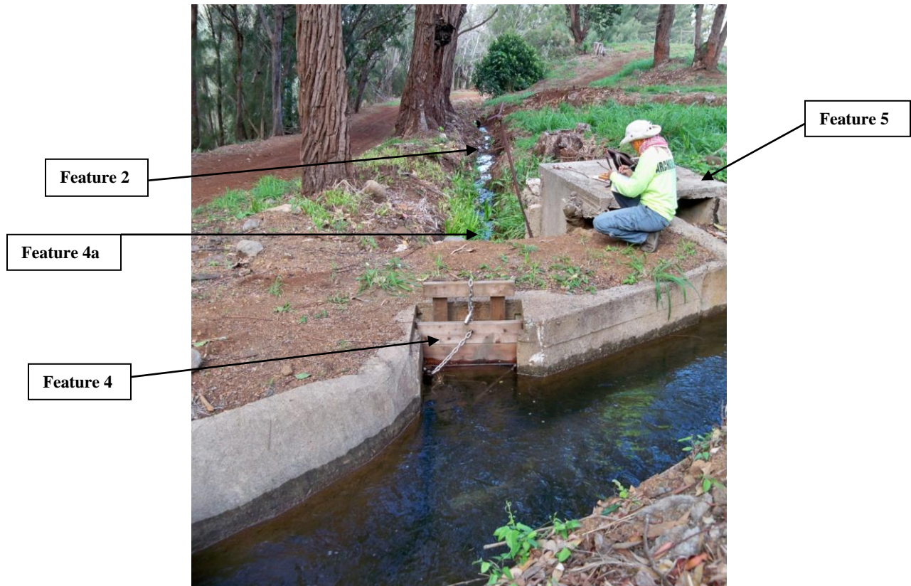
Figure 31. Photograph of Site 7881 Features 1 and 2 ditches and diversion structures Features 4, 4a and 5 (View to South)
