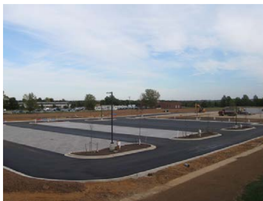
Finished parking lot
