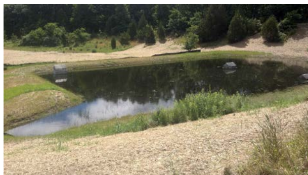
Todd Road Basin - After
