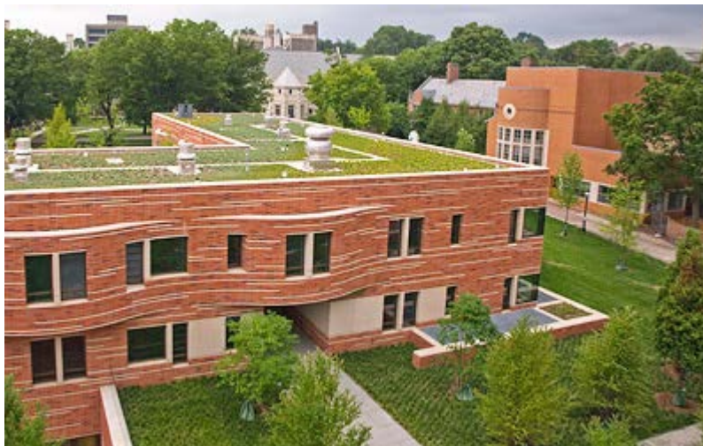
The green roof on Dormitory A is viewed here from Dormitory D. (Photo: Brian Wilson)
