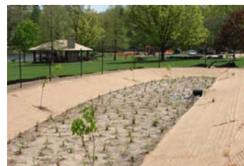
After plant and soil erosion control fabric installation
