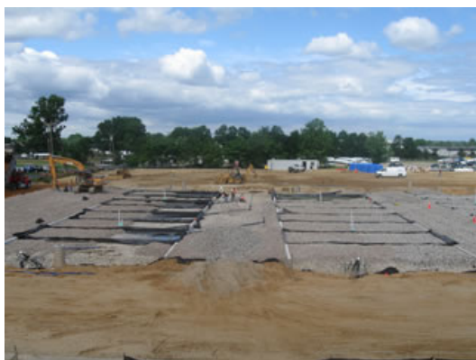
Parking lot under construction
