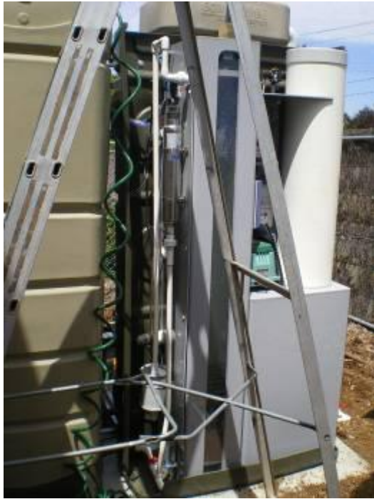
Photo 6: Installation of the prefabricated greywater system
