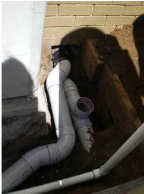
Photo 3: Laying the pipes
