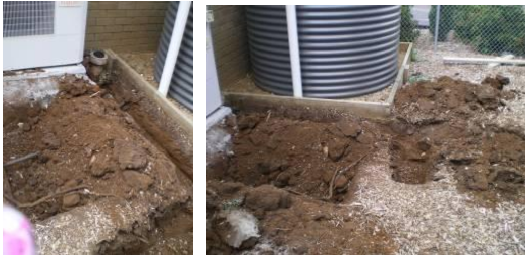
Photo 1 & 2: Digging the trenches for the pipe work.
