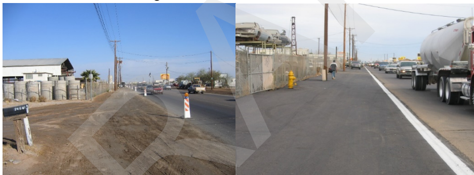
Before and after of surface stabilization on the shoulders of Broadway Avenue.
