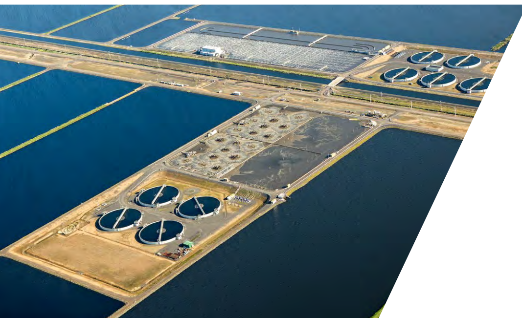
Western Treatment Plant – activated sludge plants within the treatment lagoons have enhanced nitrogen removal. Photo - Melbourne Water
