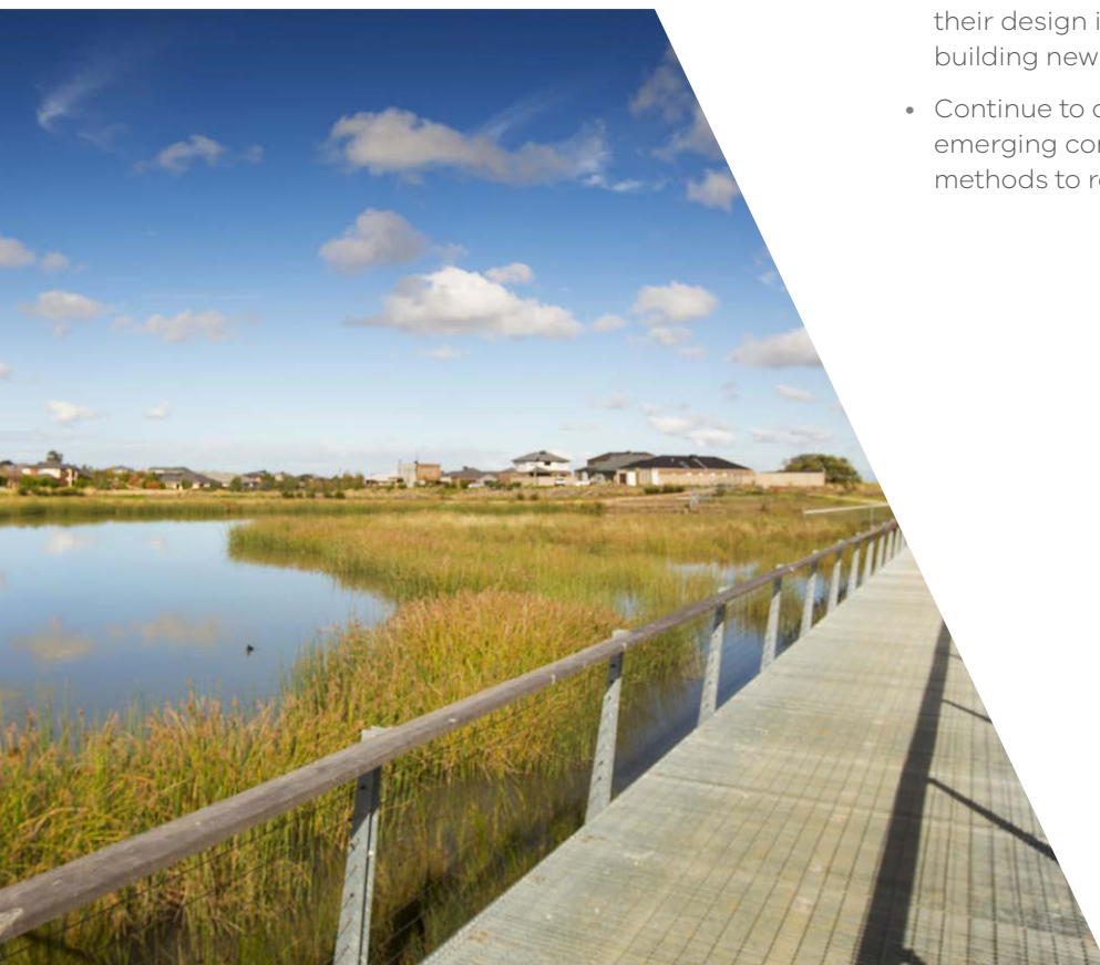
Constructed wetlands require regular maintenance to ensure that they remove nutrients, sediments and other pollutants from stormwater. Photo – Melbourne Water
