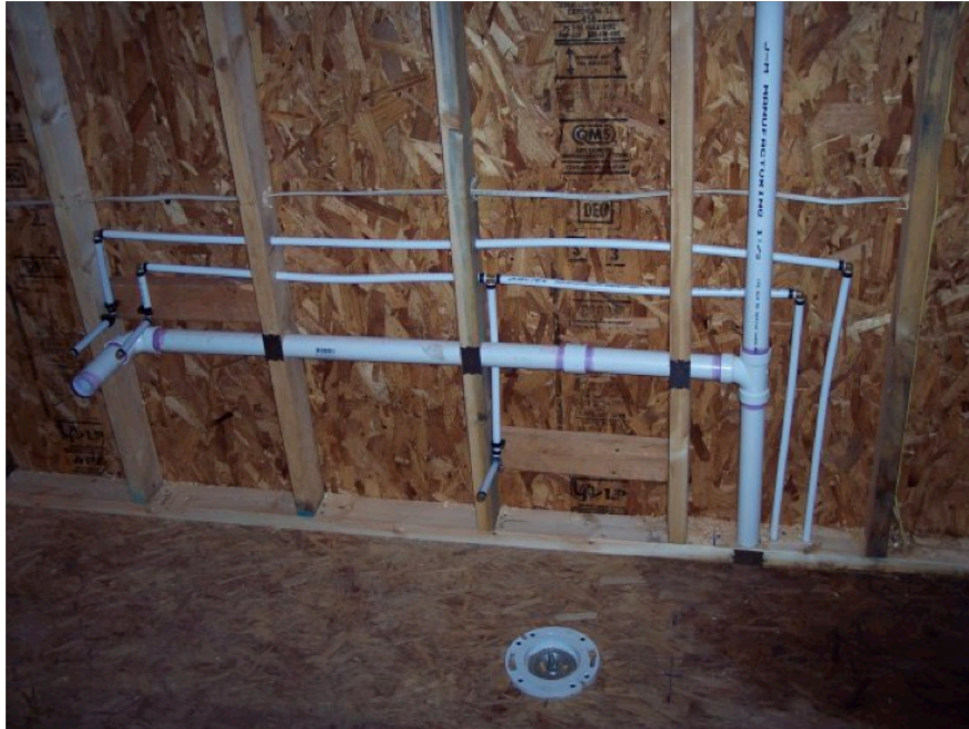
Figure 24—Drainage and water lines
