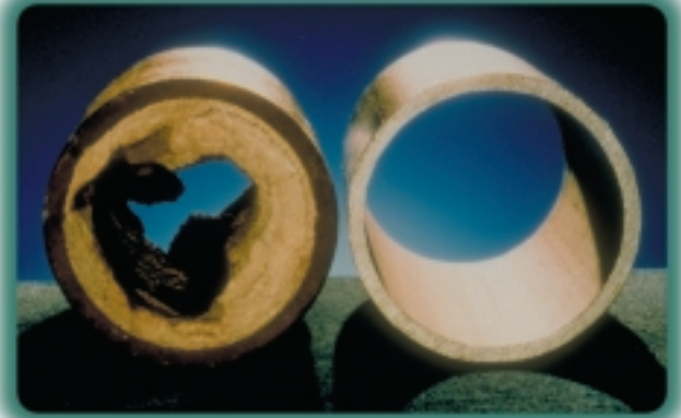
Increasing accumulations of sludge deposits in boiler tubes mean larger reductions in heat transfer capacity and boiler efficiency—and scale build-up, shown above, has a comparable effect. Cleaning or replacing blocked tubes adds direct costs.
