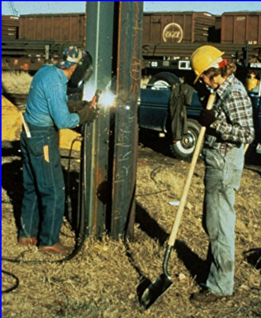
Full Penetration Groove Weld
