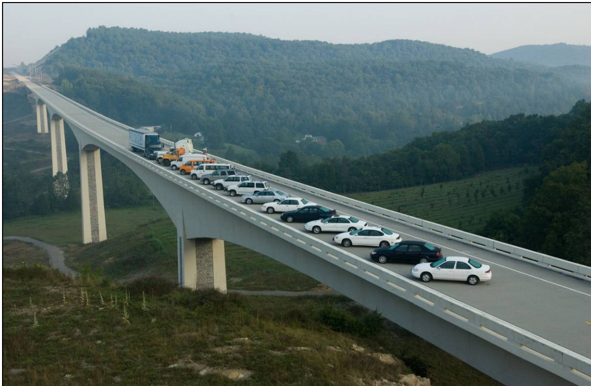
Figure 63. VTTI's vehicle fleet on the Smart Road bridge.
