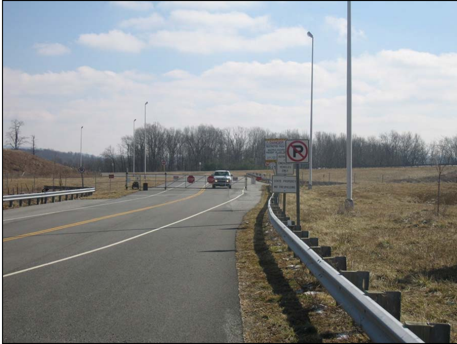
Figure 61. Gate that restricts access to the Smart Road.
