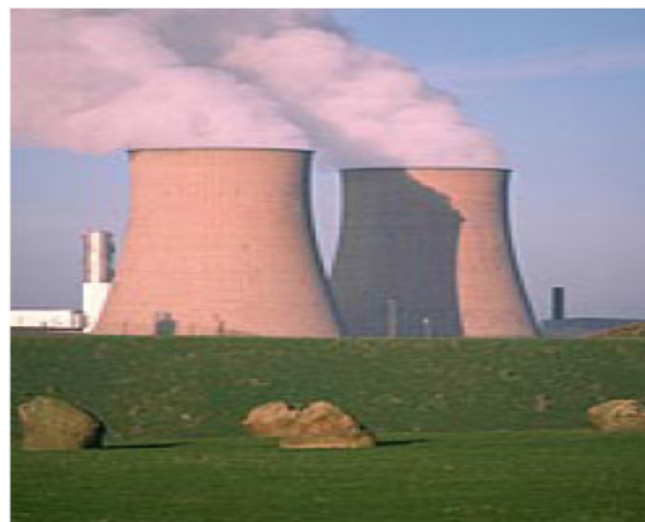
Fig.4 Natural draft wet cooling tower in power plant
