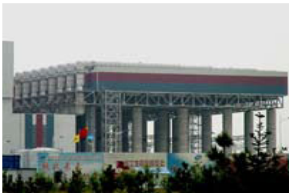
Fig.3 Zhenglan Inner Mongolia Province — ACC for 4 x 600 MW Coal Fired Power Plant
