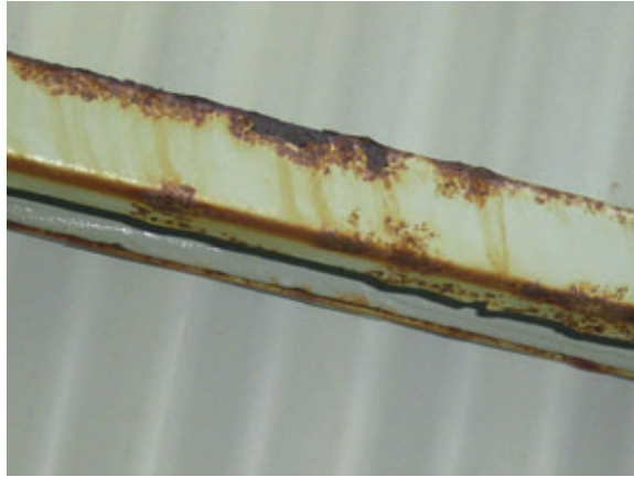
Fig. 4: Coating breakdown at an edge
