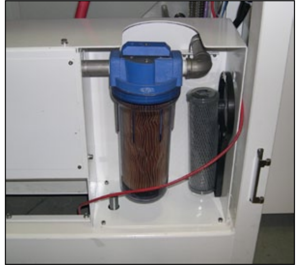
Figure 66. Inspect Water Filter Monthly and Replace Filter as Necessary.
