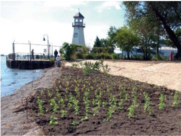
As a result of our commitment to the environment, we have transformed a 200-foot expanse of concrete and metal at our River Rouge Power Plant into a naturally sloped haven for birds, animals and visitors.
