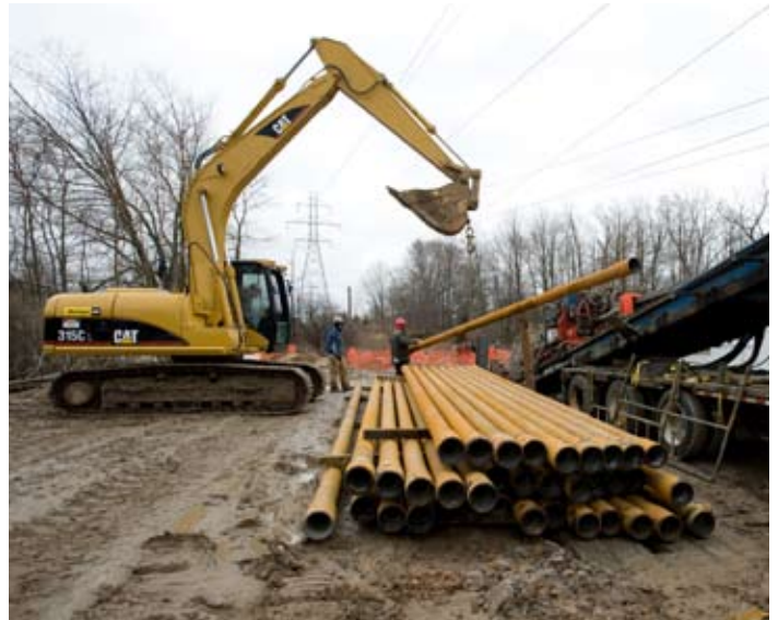
Construction on the Jamestown Pipeline in Western Michigan.
