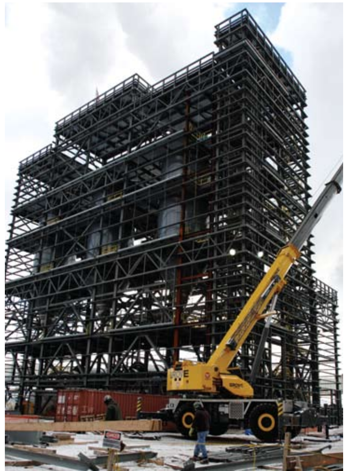
Flue gas desulfurization equipment, commonly known as scrubbers, controls 95 percent of the sulfur dioxide emissions at our power plants.
