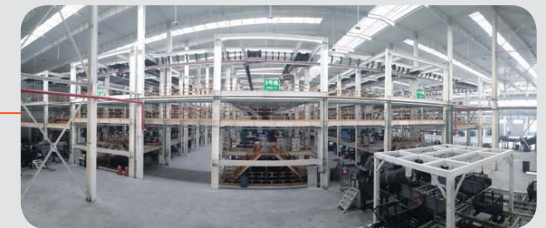
Threading, Air Pressure Test, and Anti-rust Treatment
