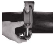
5. Housing installation
