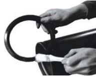
2. Lubricate gasket
