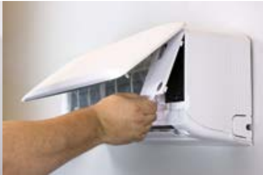
Remove electrical access panels (2)
