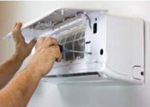
Back out electrical panel screws
