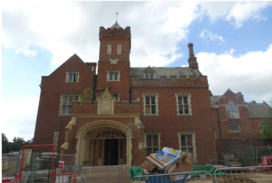
The Frythe Under reconstruction 2015
